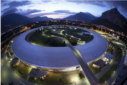
A synchrotron is a truly gigantic, stadium-sized machine that produces multiple beams of X-ray light. The machine uses different magnetic fields and radio frequencies to keep electrons accelerated at almost the speed of light in a ring tube maintained under high vacuum. This results of the production of X rays around the ring.
